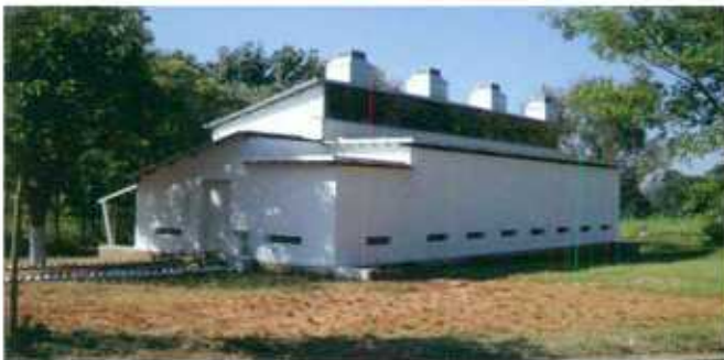
Figure 1: A view of the solar passive silkworm rearing house in the campus of SSTL, Bengaluru
