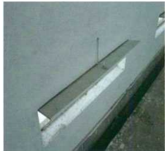
Figure 3: Ventilators provided with shutters to operate appropriately in different seasons
